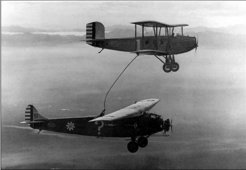
The first sustained test of air refueling occurred in 1929 when the flight of the *Question Mark* stayed airborne for more than 150 hours across 43 in-flight refuelings. Note the hose being held by an occupant of the receiving aircraft, possibly Maj. Carl Spatz (the spelling later changed to Spaatz).
